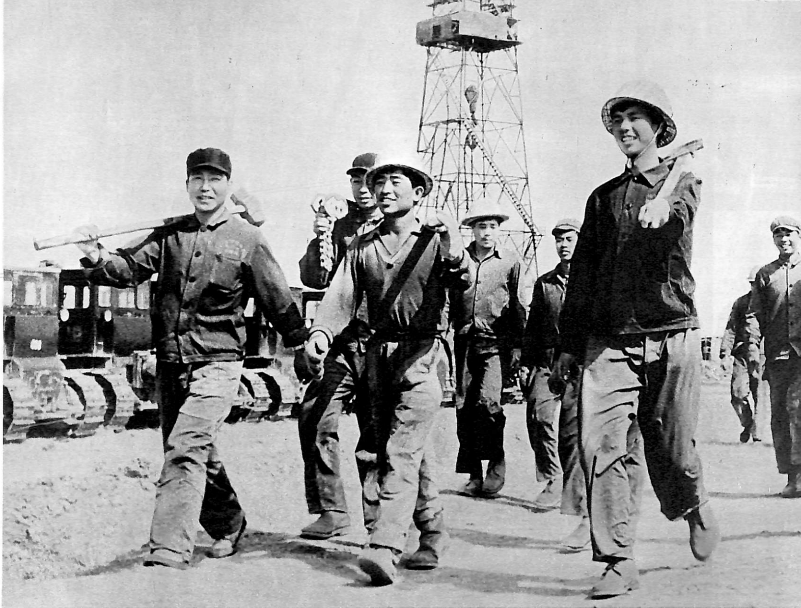
Workers of drilling team 3227.
